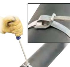
5) Using flathead screwdriver, bend retaining tab down and over cut end.
