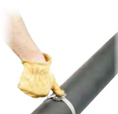
4) Remove tool, press cut end down toward retaining tab.
